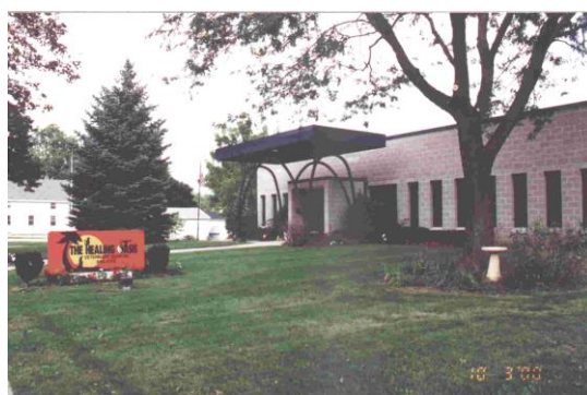
School building – picture above
