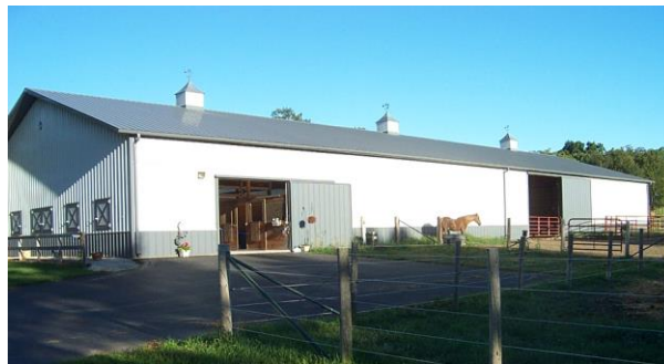
One of the private facilities used by the school
